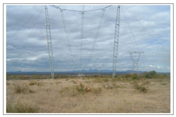
Figure 31 Eskom's existing 400kV power lines constituting Corridor 08 between the N11 and the Witkop Substation (above).
